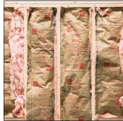
R-13 Batten Insulation In Walls & Ceiling
