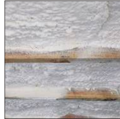
R-13 Closed Cell Spray Foam Insulation In Floor
