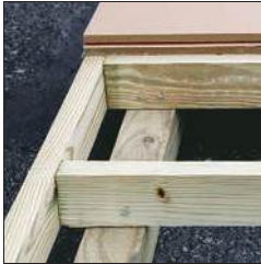
Pressure Treated 2x4 Floor Joists 4x6 Runners
