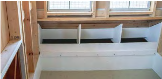
Our Deep Litter Option has 12 in. high non-porous Azek panels to prolong coop integrity and make clean out easy.
